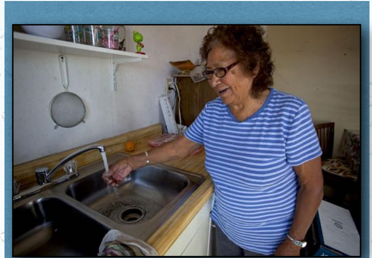
A woman tries out a newly-installed faucet in her home on the Navajo Nation. The Navajo Water Project installs self-contained water systems that include a sink, a cistern, pump, heater, and plumbing.
